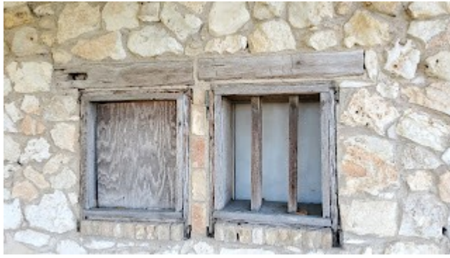
Window lintels are hand hewn, may have been repurposed from older building.
