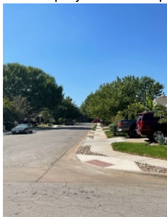
Austin's Colony R.O.W. Improvements project
