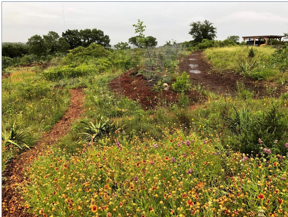
Vireo Preserve bioswale 6 months following installation (May 2020)
