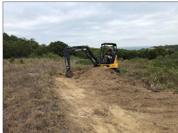
Installing Vireo Preserve bioswales, using a laser level to align on contour and digging with mini-excavator
