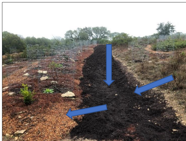
Vireo Preserve bioswale, showing direction of water movement and infiltration
