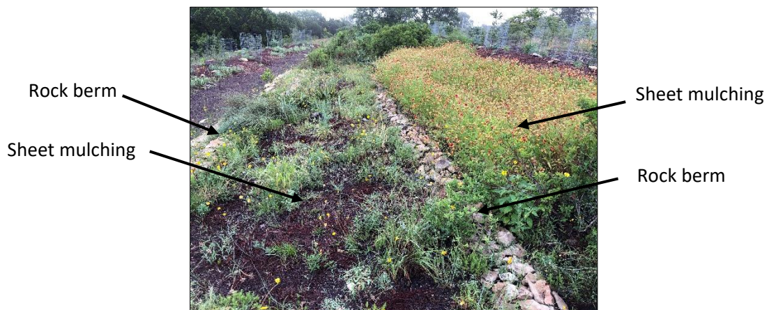
Two rows of rock berms and sheet mulching
