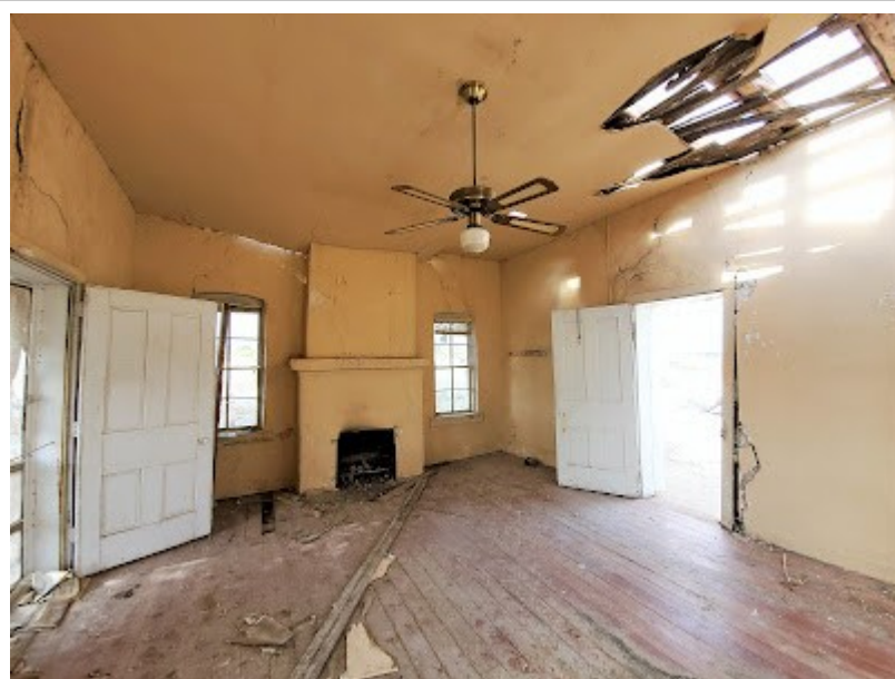
Interior looking to fireplace on West wall. Notice internal chimney, not attached to exterior.
