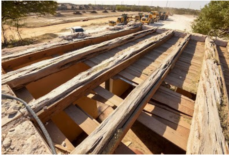
Massive cedar beams of roof. As with the Wieland blockhouse, from mill on Bull Creek?
