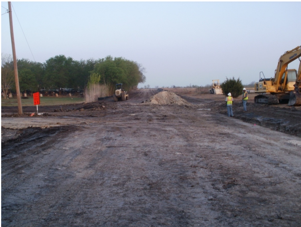
Lava Lane During Construction
