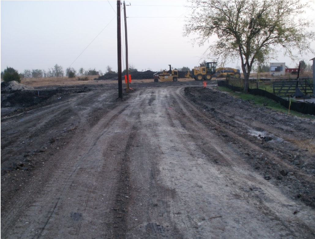
Lava Lane During Construction
