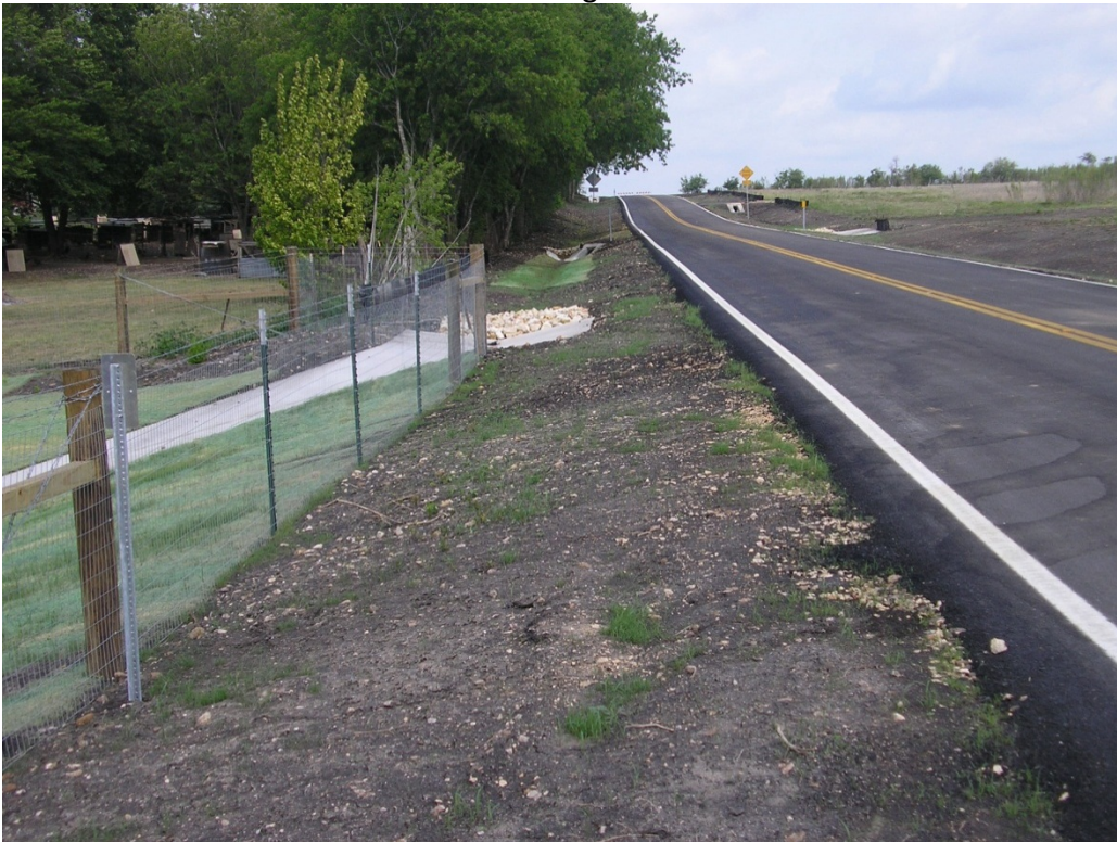
Lava Lane at Project Completion
